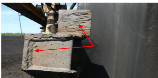
c) Detail that indicates the cause of geodesic deviation of parent material during the repair of carrying structure;
