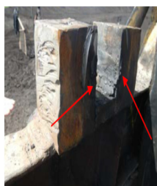
e) Damage at the carrying structure of an embedding of the stacker conveyor rejecting drum – side view;
