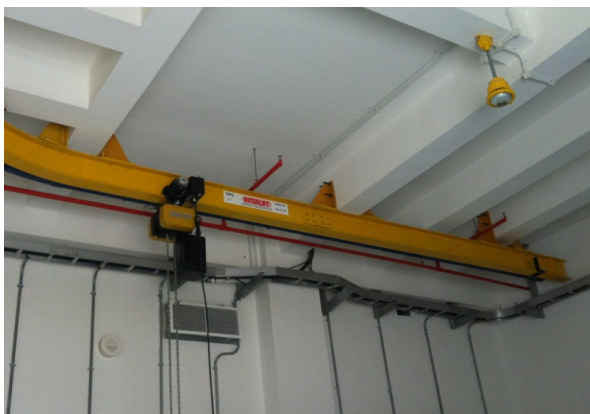
Figure 1. Runway beam for hoist with trolley
